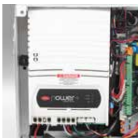
Built-in variable frequency drive.
